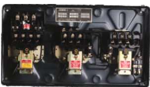
Interior View of MK1 FASD
