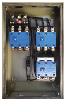
Interior View of ML FASD
