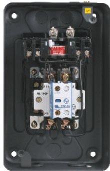
Interior View of MU-2P DOL Starter
