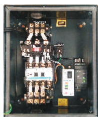
Interior View of MU-G10W DOL
