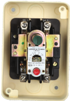
Interior View of MF1 DOL - 1Ø Starter
