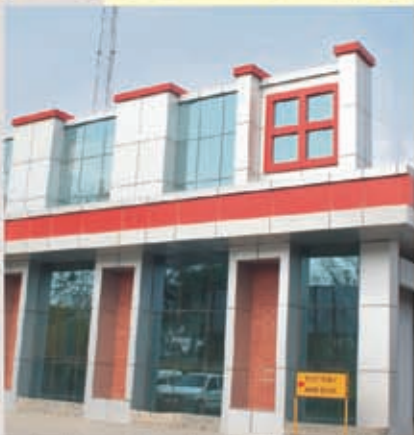
Faridabad: Industrial Switchgear Plant
