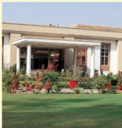
Sahibabad: Industrial Switchgear Plant
